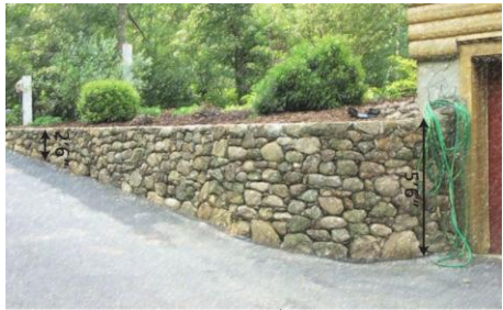
Figure 3-04. Retaining Wall Height
